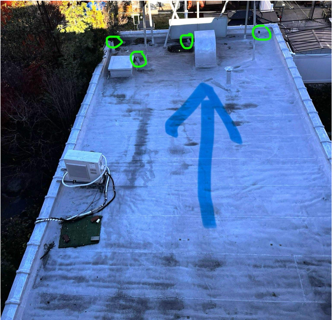
Pipes that could be covered.
